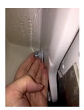
When changing the basin in the future. Just remove the old basin, loosen the screws, adjust the bolts to the corresponding distance of the new basin, retighten and re-fit.
