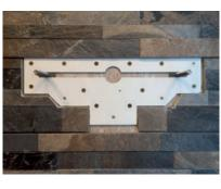
**5.** Put silicone on the back of the wash basin where it meets the tiles, this will help reduce noise vibration. Offer up the wash
