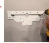
**4.** Once the plate is in position tile around and up to the edge. The plate can be installed on a pre-tiled surface. the Wash basin will stand proud of the wall by 3.8mm but this can be siliconed.
